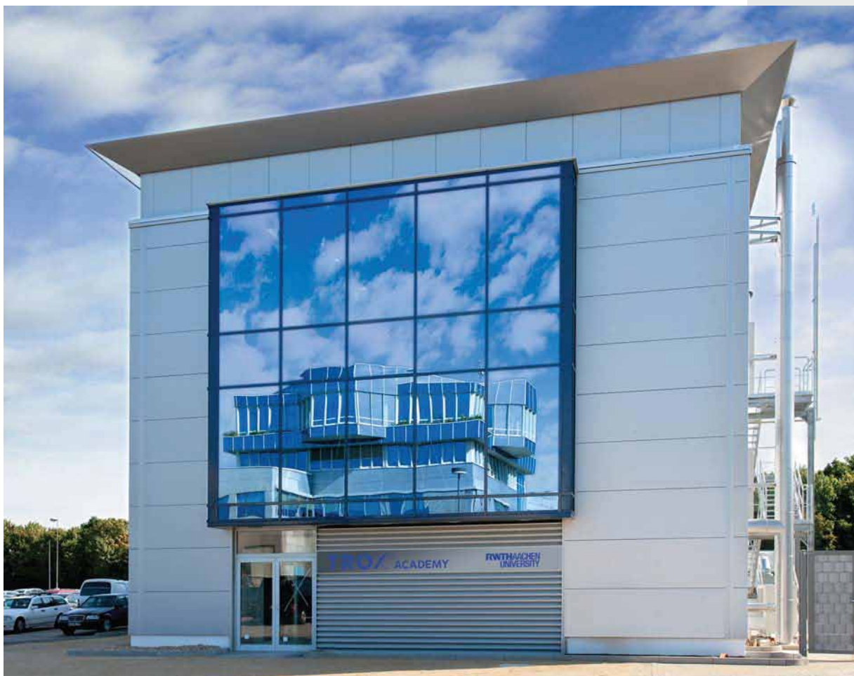
The International Center Fire Protection (ICB) in Neukirchen-Vluyn, Germany, opened in 2009.
